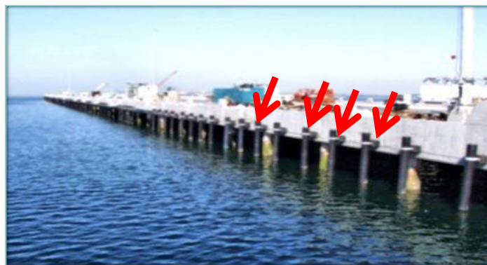
Fig 1. FRP wrapped Columns as retrofit for bridge (Source: Wikipedia)
